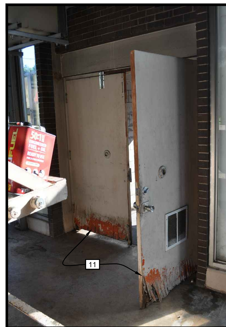
9 Interior Door at Bottom of Tower New Infill with Storefront Framing
