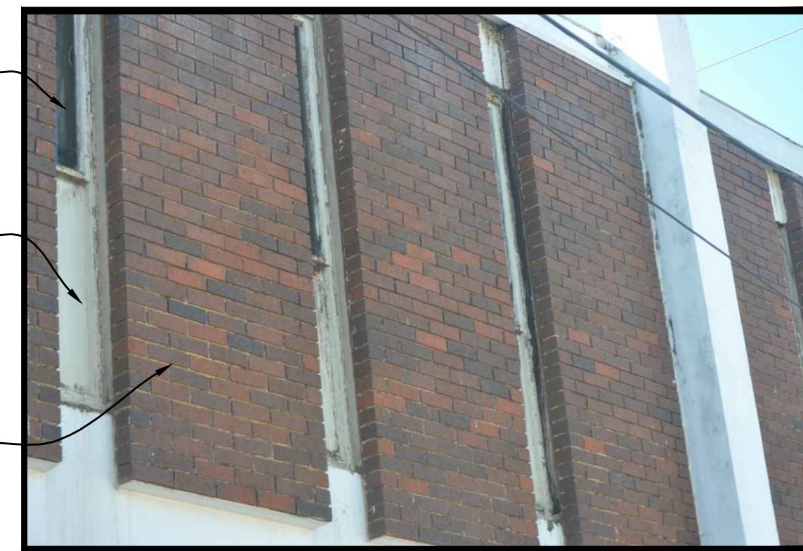
2 Partial View of Second Story Facade Steel Framed Windows and Panels
