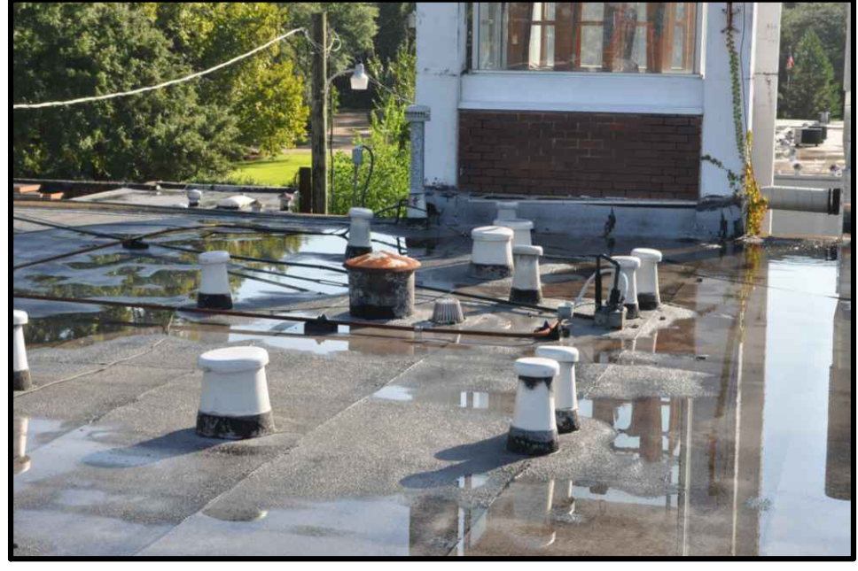
P8 Roof Penetrations (Looking North To Tower)
