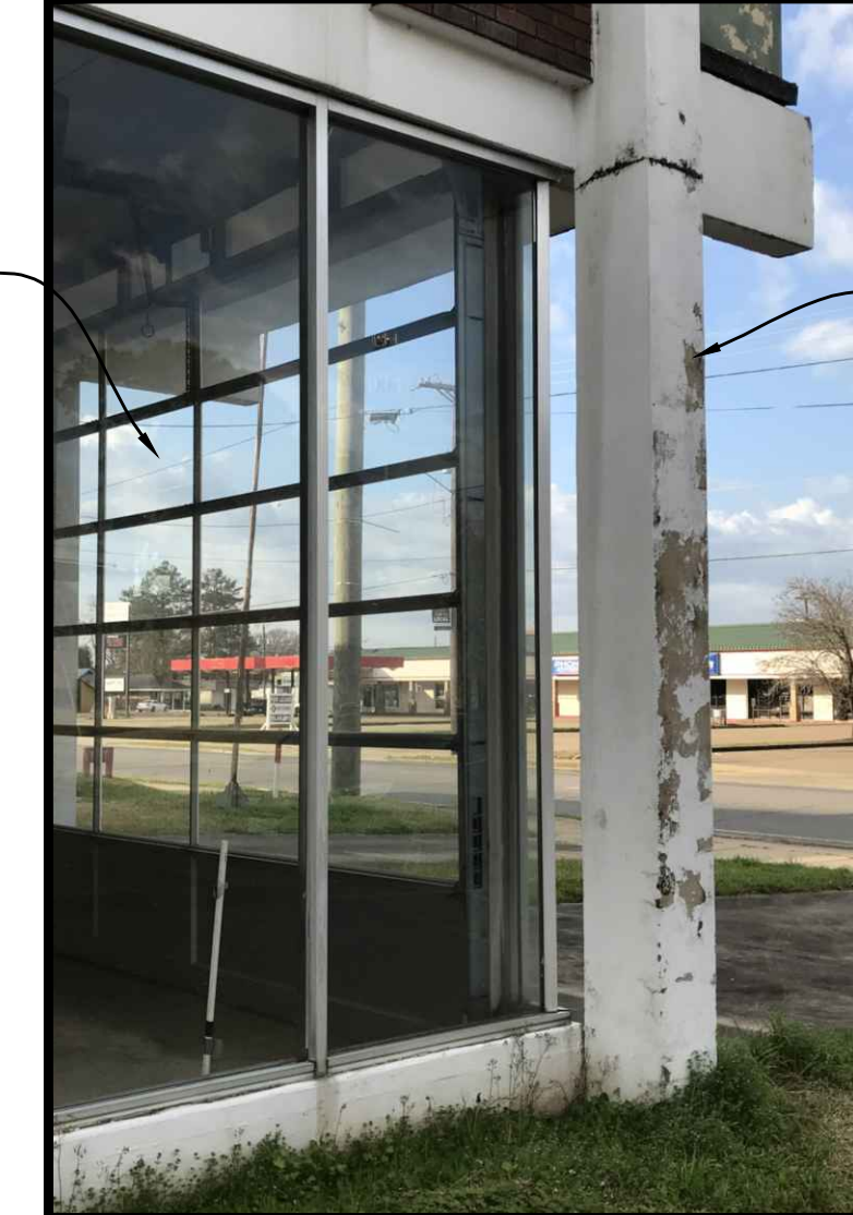
8 Building Corner South West Corner at Texas Ave.
