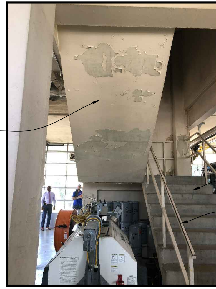
2 Stairway First Floor
