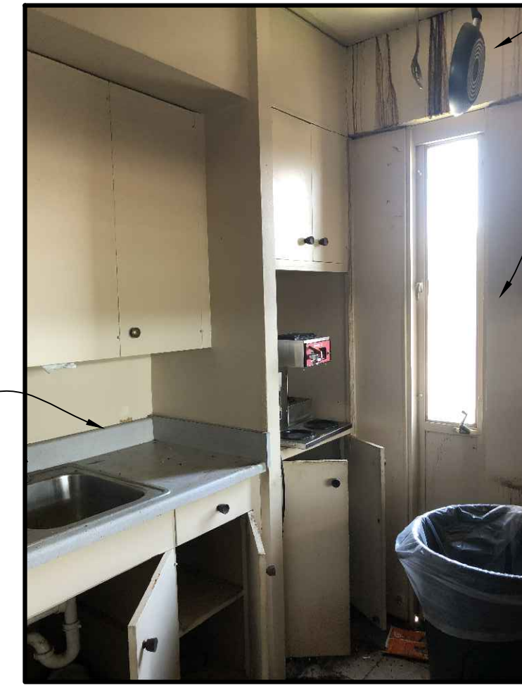
10 Second Floor Kitchen
