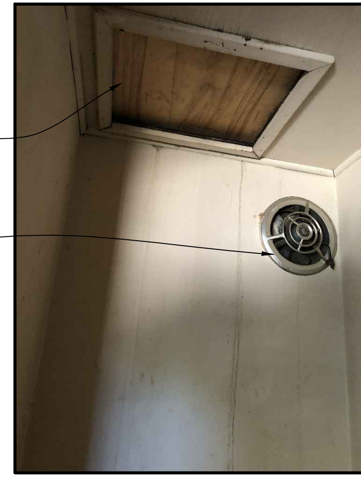
5 First Floor Toilet
