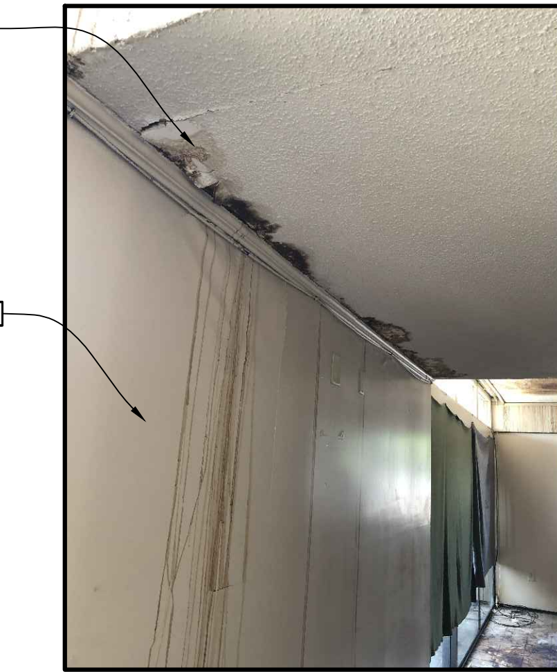
17 Second Floor Corridor
