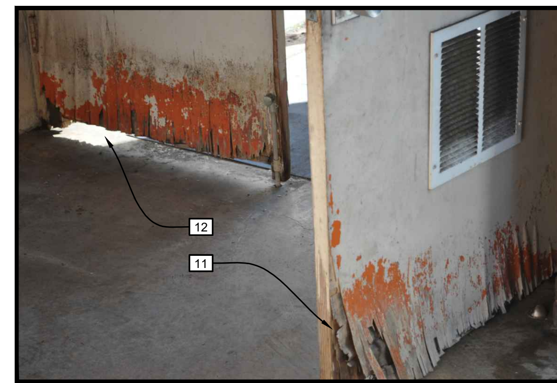
10 Close Up of Interior Door at Bottom of Tower
