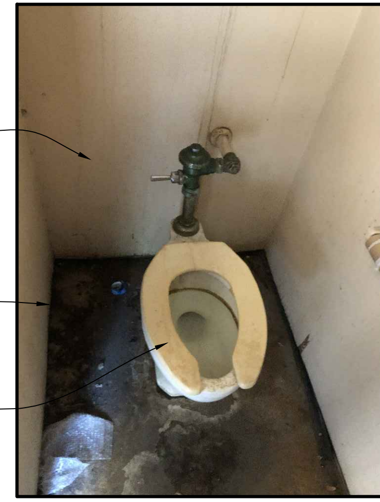
6 First Floor Toilet
