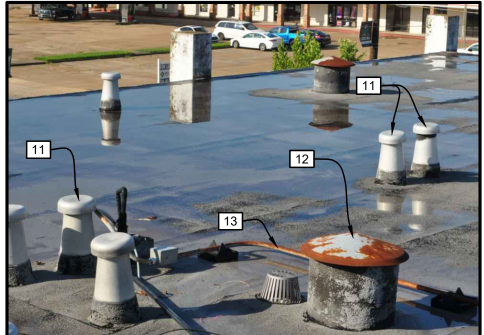
P7 Roof Drain (Looking Southeast)
