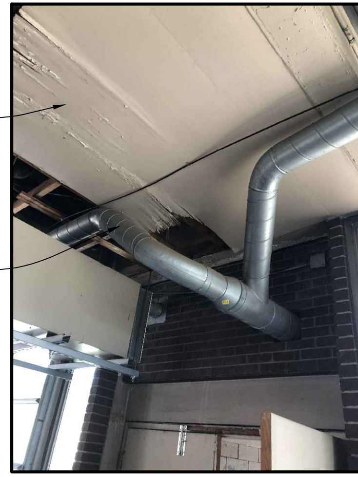
4 First Floor At Tower Doors
