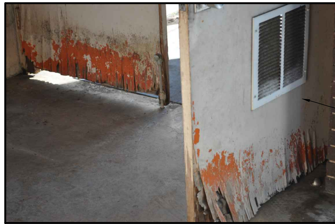
7 First Floor Tower Doors
